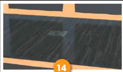
14 The shower base is finished and can be tiled.
